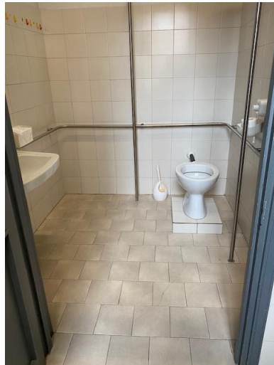
Bagno piano terra
