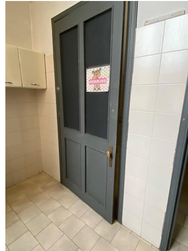
Bagno piano terra
